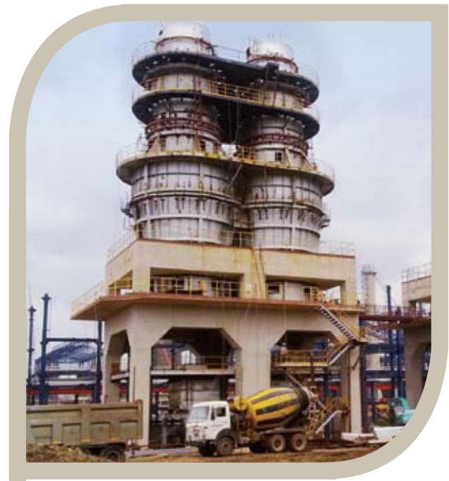
Greenfield project – Kiln 2, Odisha, India
